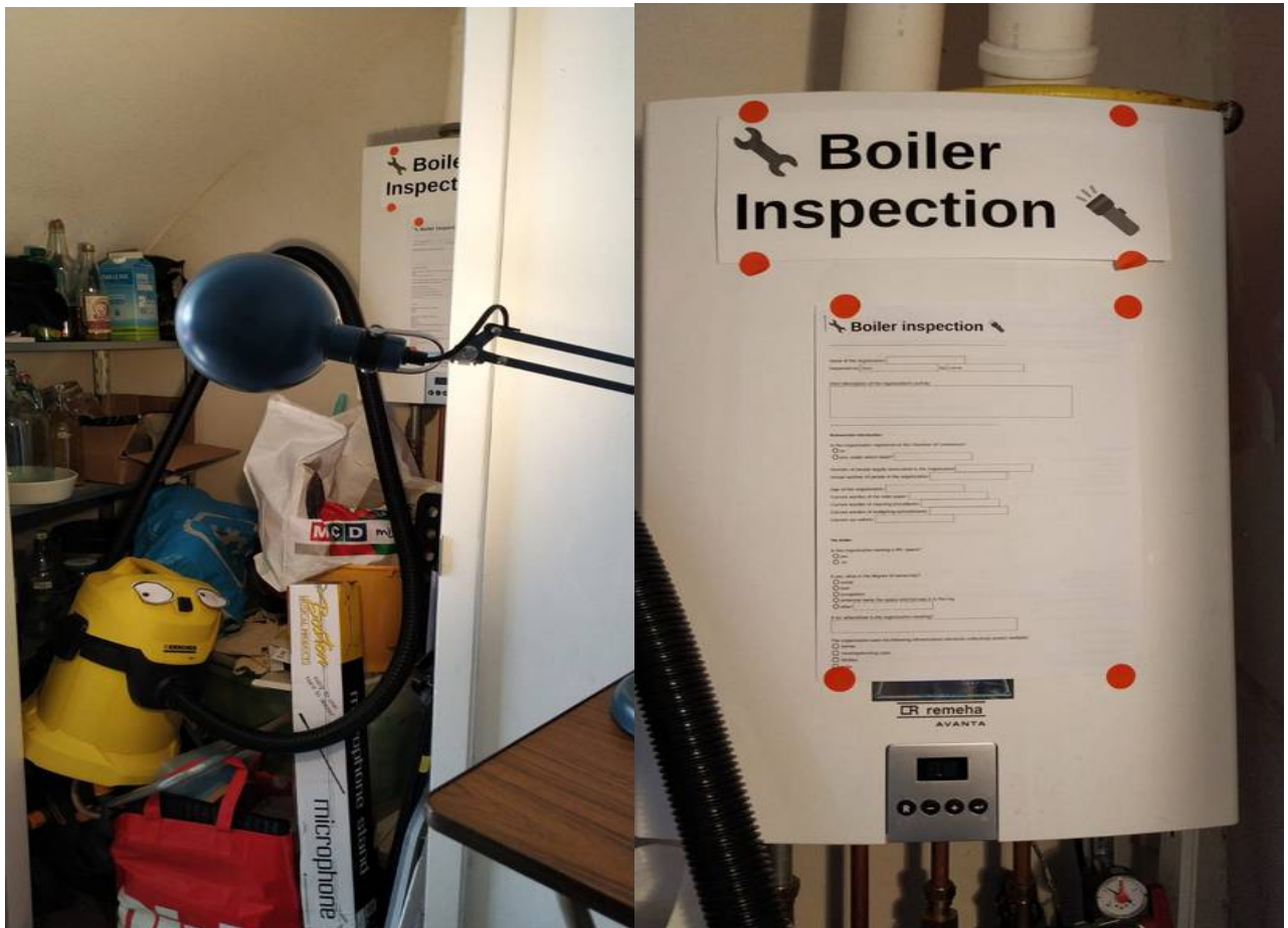
Figure 5: Boiler inspection at Varia
